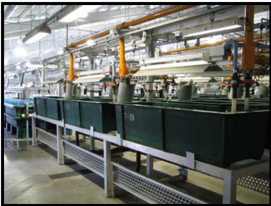
Figure 9. Tanks utilized for feed training Florida largemouth bass fingerlings.
