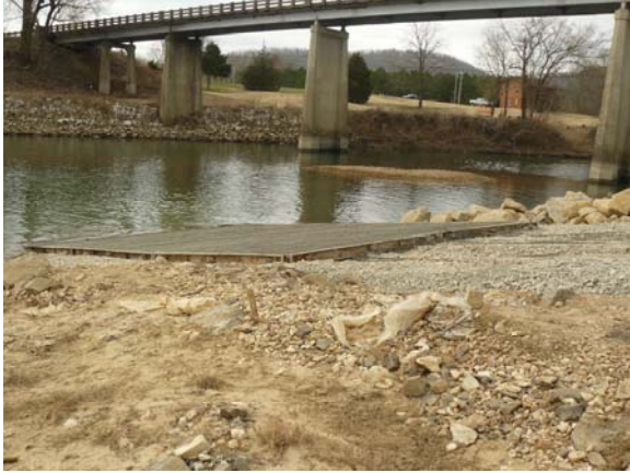
New Sylamore Access boat ramp while under construction
